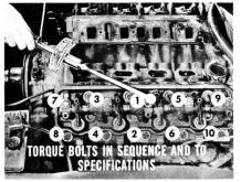
After you install the heads, rocker arm brackets and arms, use a torque wrench to tighten the head bolts in their proper sequence. After you've drawn down each bolt to 50 footpounds, go around again and pull them down to the final torque specifications, 70 footpounds on this engine.
